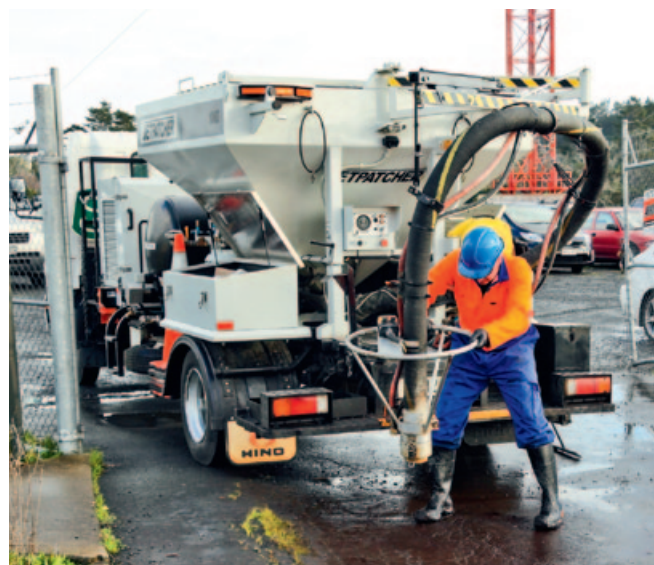
Jim (at left) and Scott Turnbull. Jim developed the Jetpatcher process during the 1990s and has now exported over 500 machines. Below: Filling a pothole is a quick one-man operation.
